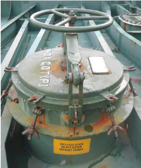
Figure 3: COT No. 1P access hatch showing warning label.
