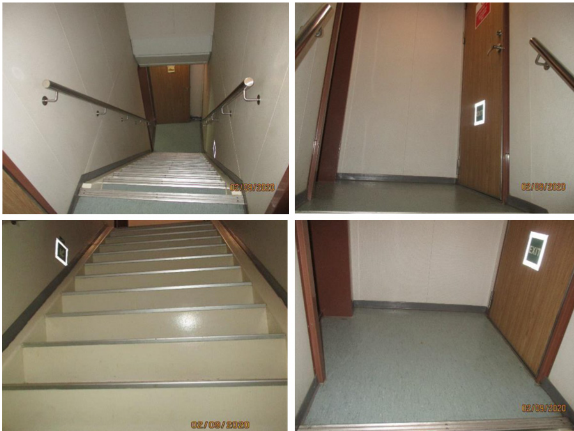
Figure 1: Stairs between the B deck and the Bridge of TIGRIS.
