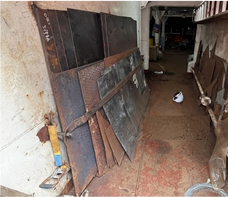
Figure 3: Steel plates stored inside of the Forecastle Store. The ASD1's safety helmet is lying where it was found after the incident.
