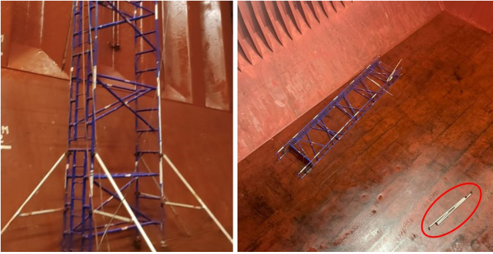
Figure 4: The photograph on the left shows the scaffolding in use previously on board PRISMA with all four stabilizer arms in place. The photograph on the right shows the scaffolding lying on the tank top in CH No. 3 after it fell. The two stabilizer arms that had been removed are circled in red.
