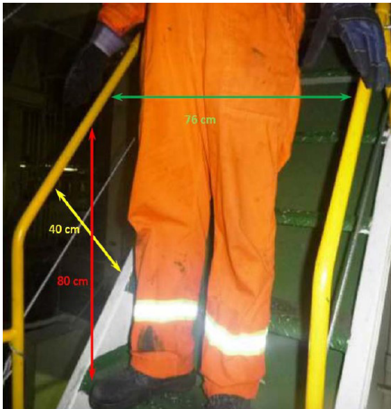
Figure 2: Dimensions of inclined ladder between the second deck of Engine Room and the upper deck. (Note: Rope which is affixed in the position of an intermediate railing was not in place at the time of the incident.)
