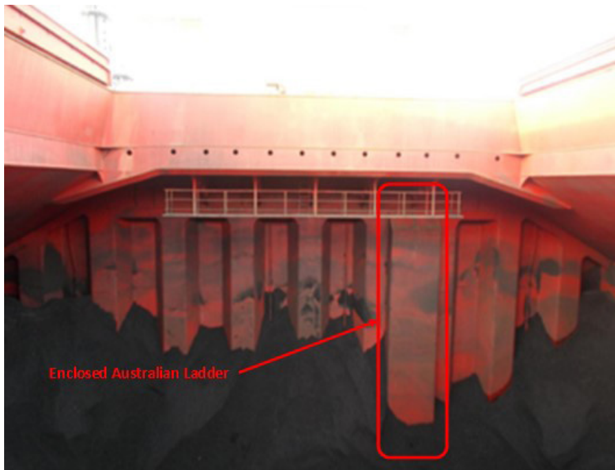
Figure 5: Cargo level in Cargo Hold No. 6 at time of entry.
