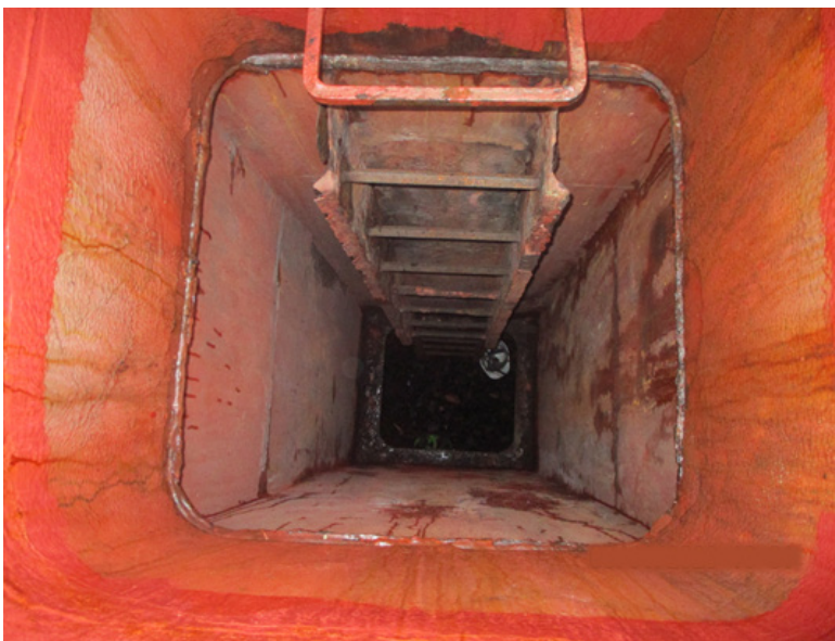
Figure 4: Photo of the aft access ladder, taken from the main deck. Note the coal in the cargo hold covering the lower section of the vertical ladder and the platform.
