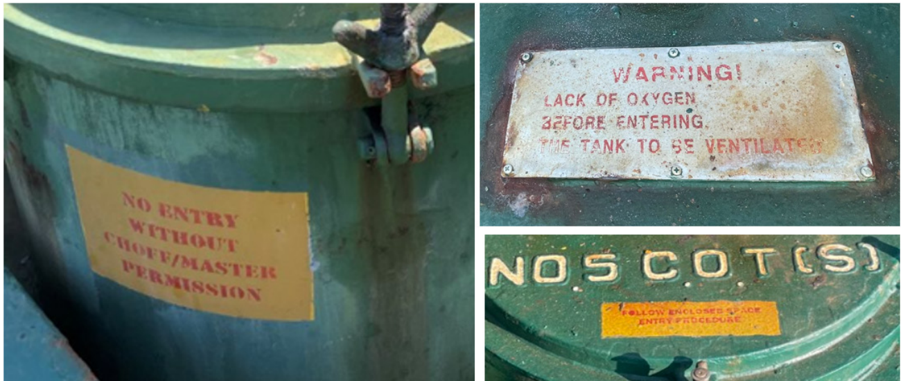
Figure 5: Warning signs located at the entrance to the access hatch to COT No. 5S.
