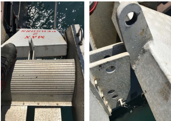
Figure 3: The lower platform of the accommodation shown as found after the ASD2 fell overboard. These pictures were taken while the ship was at anchor after the SAR operation was suspended. The securing pin had not been passed through the hole on the bar welded to the platform when it was put through the holes on the angle bracket.
