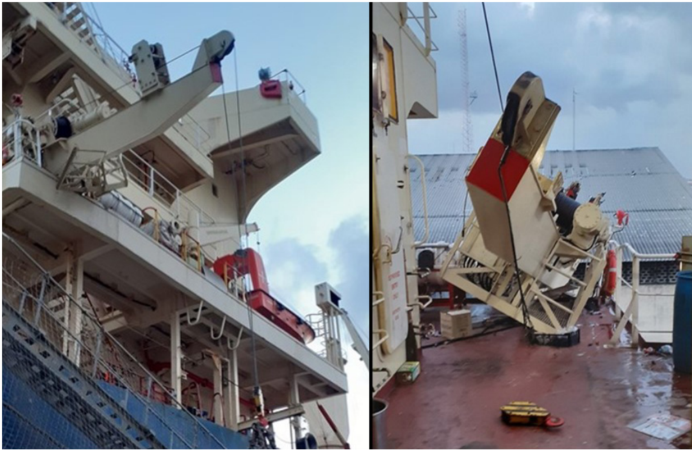
Figure 10: Photos of the provision crane following the incident.
