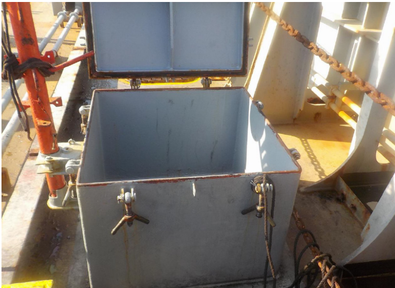
Figure 2: Sludge hatch of Cargo Hold No. 3.
