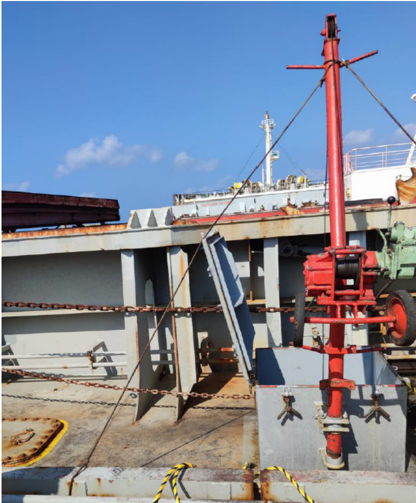
Figure 3: Mucking winch mounted over Cargo Hold No. 3 sludge hatch. Photo taken from aft, facing forward.
