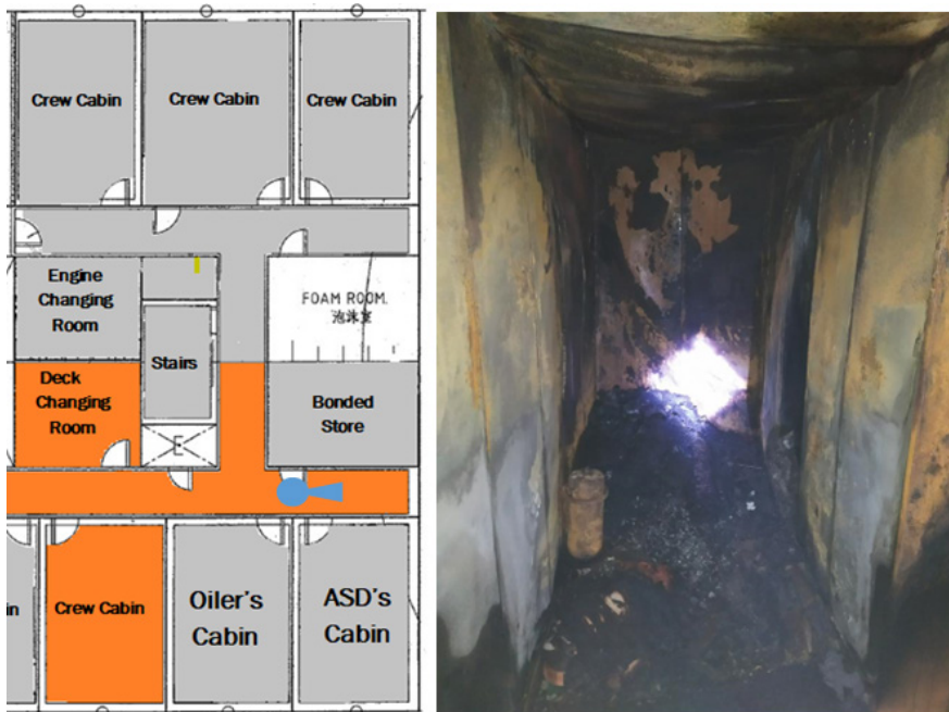
Figure 9: Photo of the passageway outside the ASD1's cabin. Orientation of view is indicated in blue.
