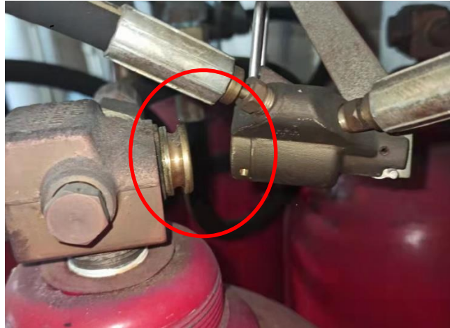
Figure 6: Pilot lines and discharge hoses found disconnected.
